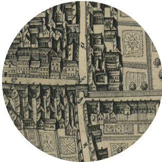
f. Cowgate Port and St Mary's Wynd Port Flodden Wall 1514 | 60
